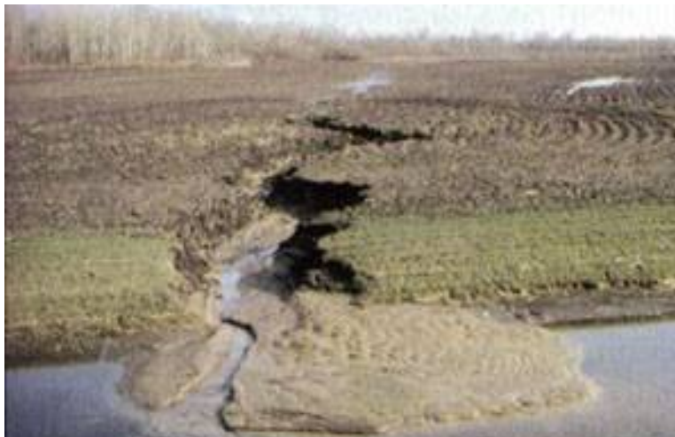
Surface water soil erosion. Courtesy of U. of Michigan.
